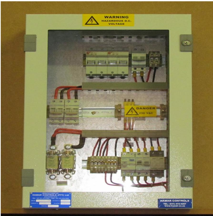
Figure 4: Solar System Distribution Board with circuit breakers
