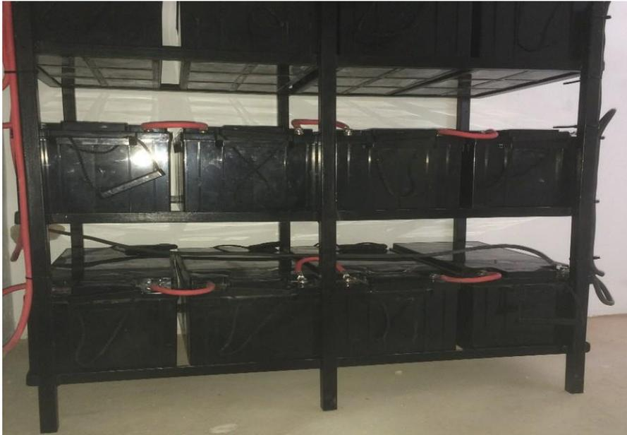
Figure 3: Battery bank with battery rack
