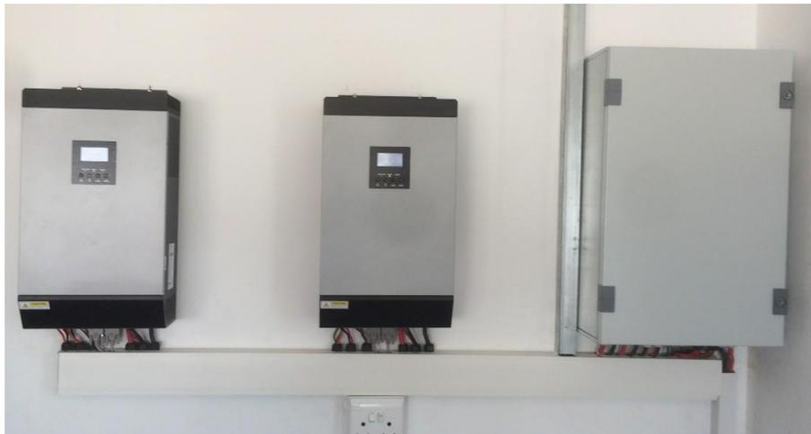
Figure 2: Inverters and Solar System Distribution Board
